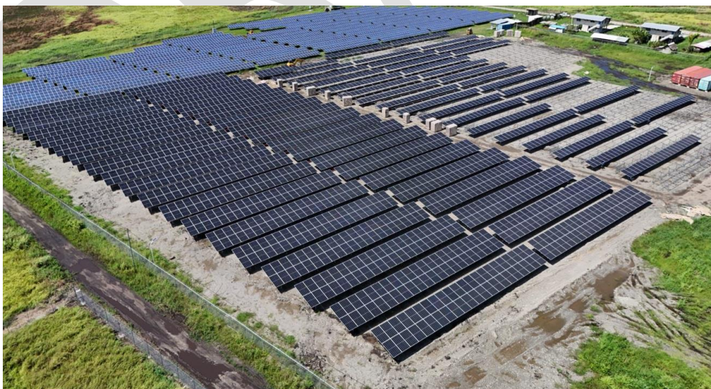
Fig. 1 Henderson 2MW Solar Farm
