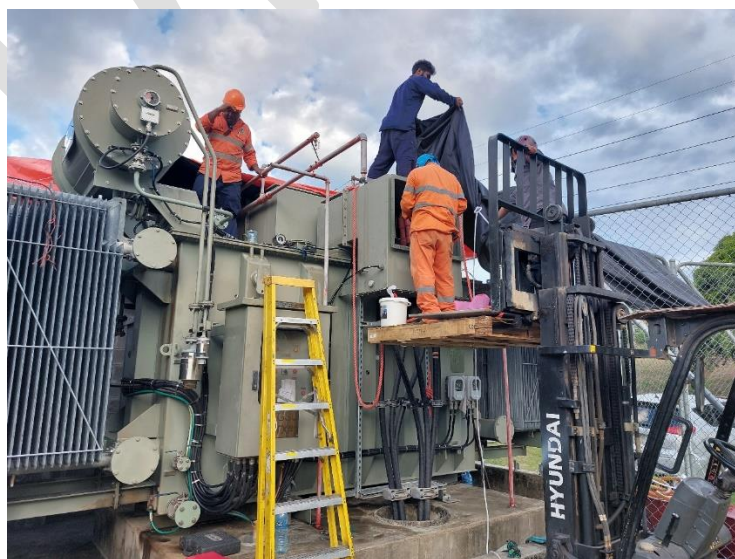
Fig 5: Repairing Power transformer at Lungga Power Station
