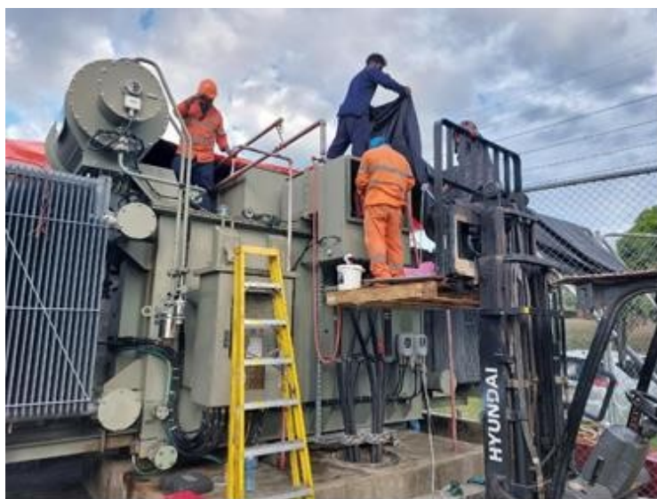
Fig 4: Repairing Power transformer at Lungga Power Station
